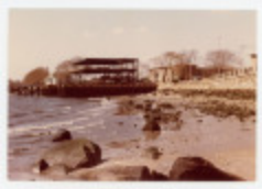
McMurray Hall Construction ()
