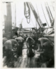
Cleaning the Deck of the St. Mary's ()
