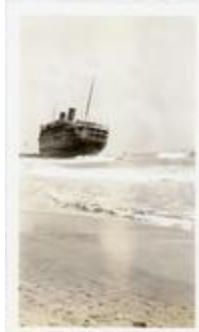
View of Morro Castle from Beach in Asbury Park, New Jersey ()
